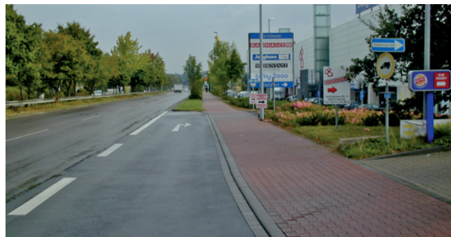
Road with turning lane to access large commercial properties
