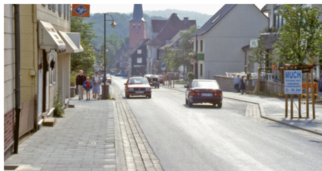
Urban main road with wide paved gutter and adapted footway space design
