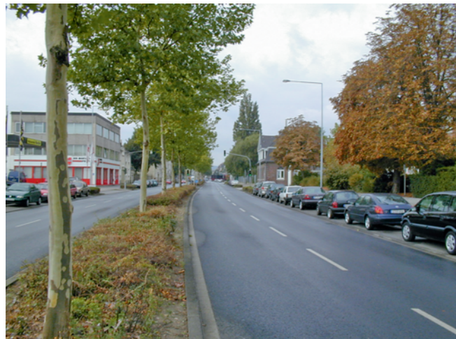
Industrial Estate road (main road) with greened central reservation and longitudinal parking lanes, also cycle paths in the footway space
