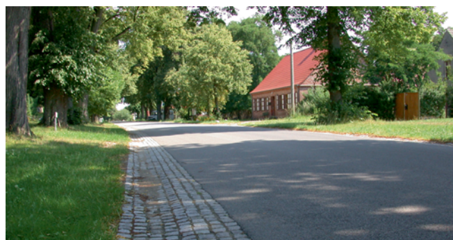
'Soft separation' between carriageway and side space
