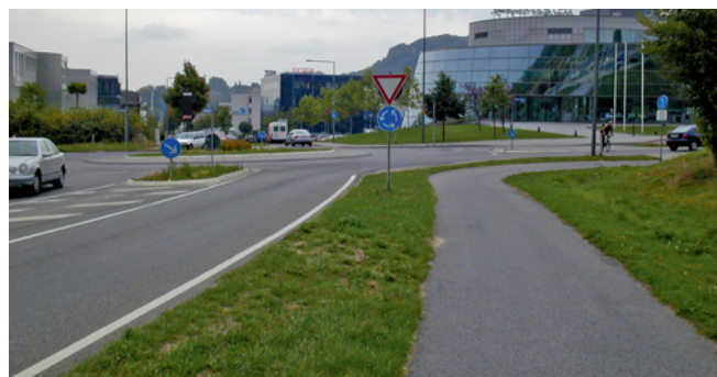
Road in a commercial area with roundabout and two-way shared footway space
