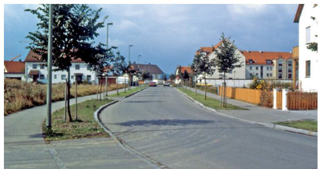
Collector road with footways behind tree-lined green border strips
