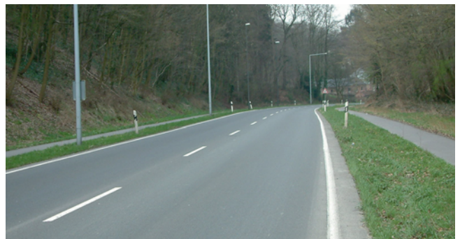
No frontage access road with pedestrian/cycle paths on both sides, approaching built-up areas
