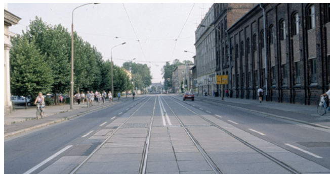
Link road with flush tram rails and 'hybrid' cycle paths
