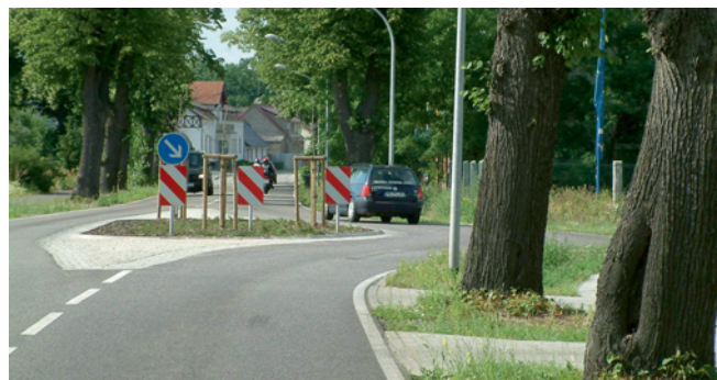
Traffic calming at the entrance to a locality using a central island with a clear offset from the carriageway
