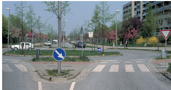
Roundabout on a collector road on a large residential development
