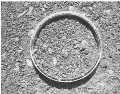
Figure 7: Ring shuttering for sealing on coarse-grained surfaces
