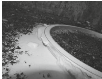
Figure 8: Ring shuttering with poured-in gypsum slurry
