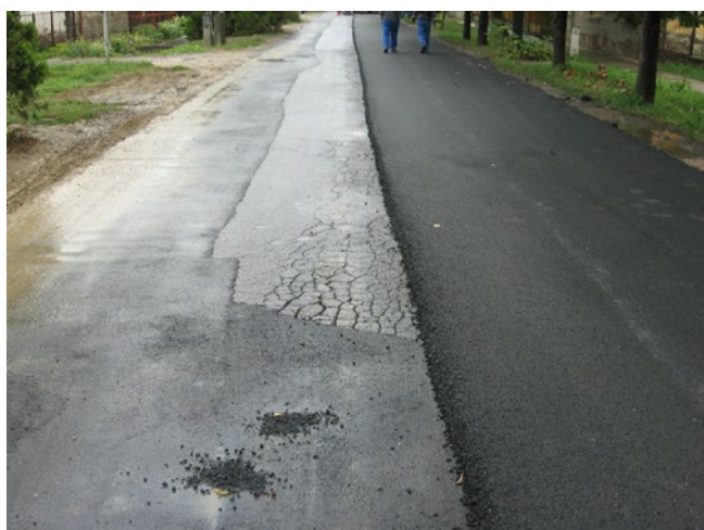
Figure 19: Alligator cracking on a surfaced base [11]
