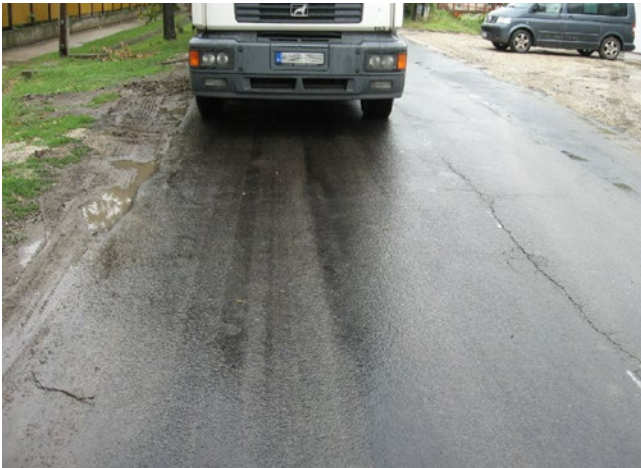
Figure 34: Base wetted by rain shortly prior to laying an asphalt surface course [11]
