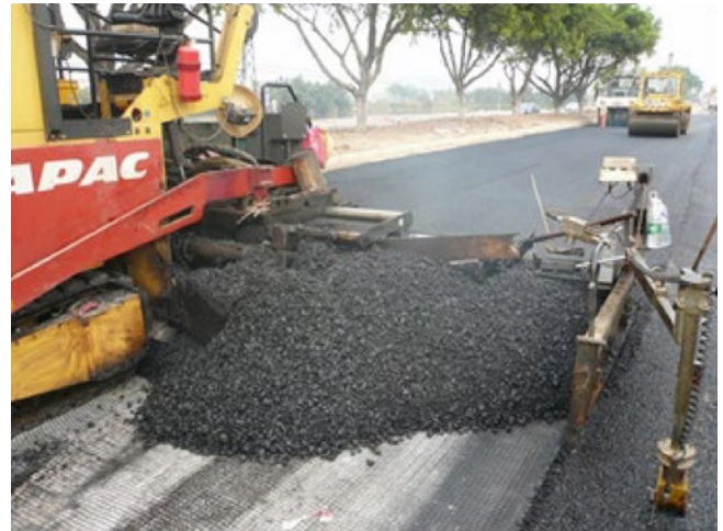
Figure 43: High material level in the left outer area of the screed and material segregation due to missing tunnel extensions and auger shaft extensions [11]
