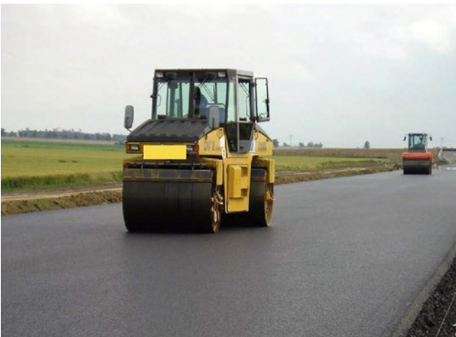
Figure 76: Use of crab steering at the end of main compaction and start of final compaction with a heavy smooth-drum roller [11]
