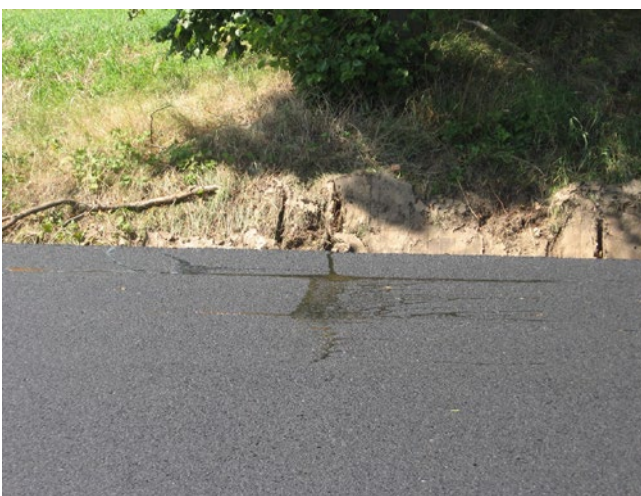
Figure 58: Trough-shaped depression in the pavement caused by a stationary roller [11]
