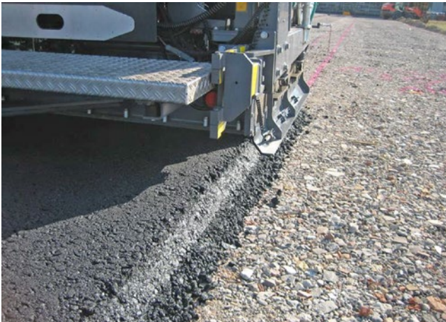
Figure 11: Paving screed equipped with an edge attachment [35]
