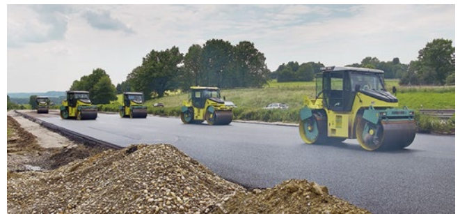
Figure 61: Adherence to the rolling areas specified by the rolling pattern [1]
