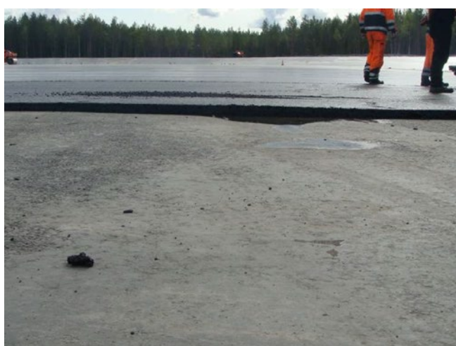
Figure 20: Height equalisation of longitudinal roughness [11]
