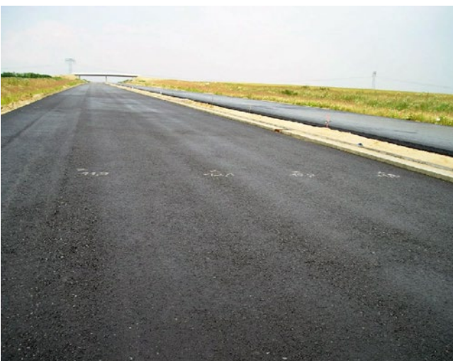
Figure 23: Marked high points on a laid asphalt base course [11]
