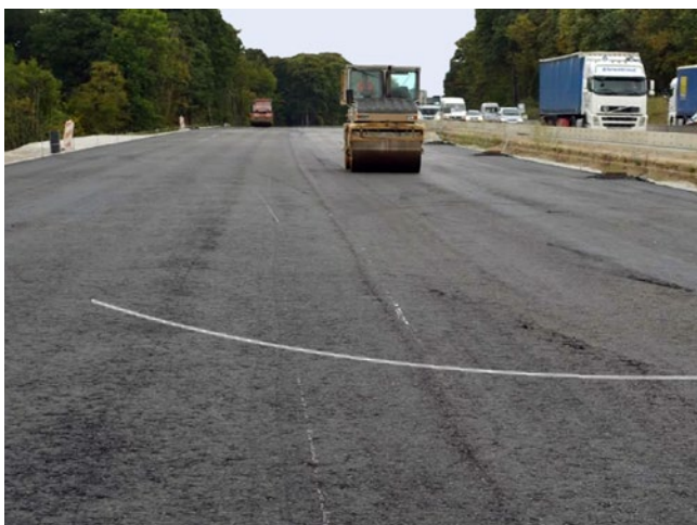
Figure 50: Two-strip "hot to hot" paving of a 10cm thick asphalt base course AC 32 T S, 50/70 with unmatched screed output (view in opposite direction to paver's direction of travel) [7]
