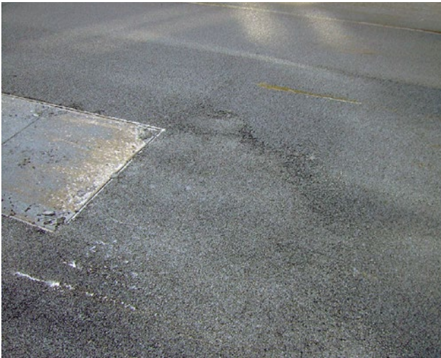
Figure 22: Incorrect overlaying of a manhole which is not at the same height [11]
