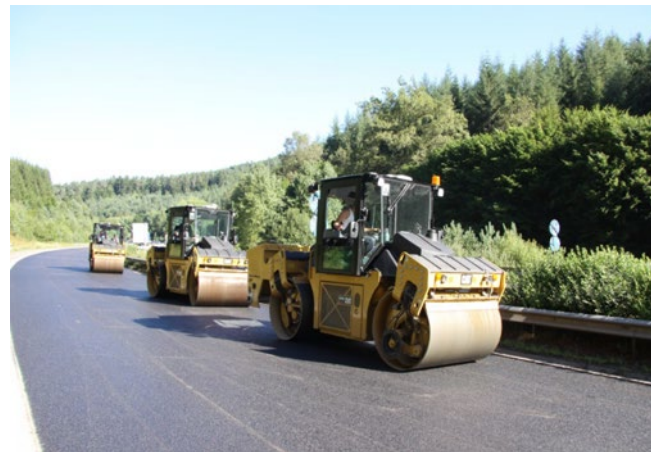
Figure 62: Adherence to specified rolling areas and keeping close together [7]
