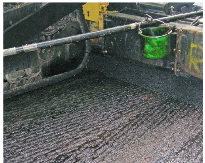
Figure 35: Paving an SMA on an incompletely cured bitumen emulsion [11]
