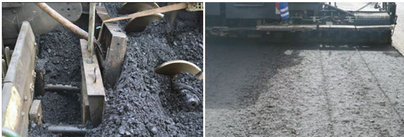
Figure 49: Cause and effect – Defective pre-strike offs cause an open structure of the asphalt course [7]
