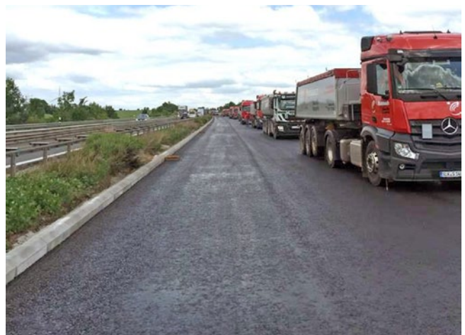
Figure 38: Long truck queues in front of paver due to inadequate transport logistics [35]
