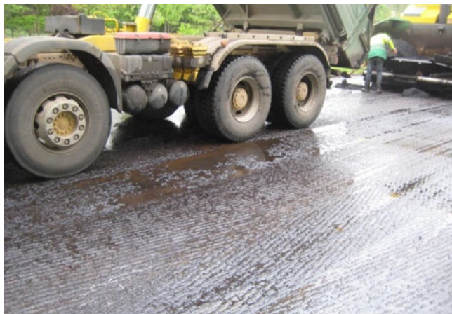
Figure 32: Joints between the milled strips and start of paving despite unbroken bitumen emulsion [35]
