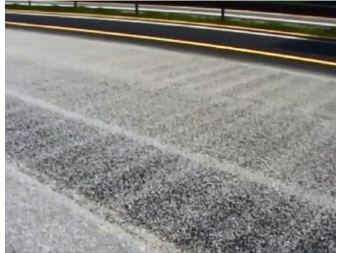
Figure 55: Short, periodic bumps in the asphalt surface course caused by an overloaded chip spreader [11]
