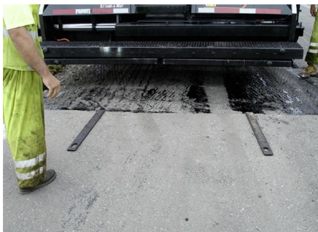
Figure 46: Use of flat steel to set the screed before paving [7]
