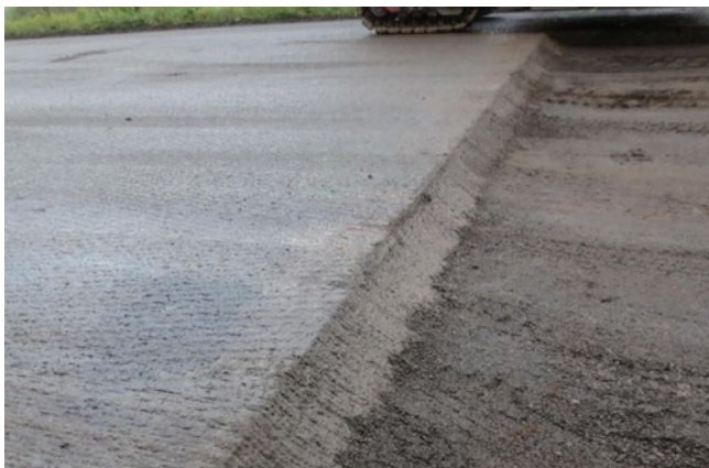
Figure 33: "Circular" connection point which was not milled or cut straight prior to subsequent laying of the asphalt base course [7]
