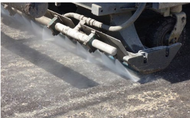
Figure 30: Cleaning an asphalt base with an unsuitable high-pressure flat-jet water spray device with upstream extraction, with clearly visible dirt remaining on the base [20]
