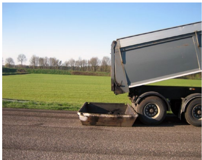
Figure 41: Good example of cleaning a truck's loading sill on-site [35]
