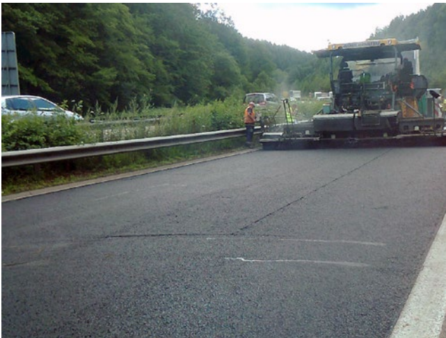
Figure 56: Cross-rolled section to reduce bumps caused by paver stop [7]
