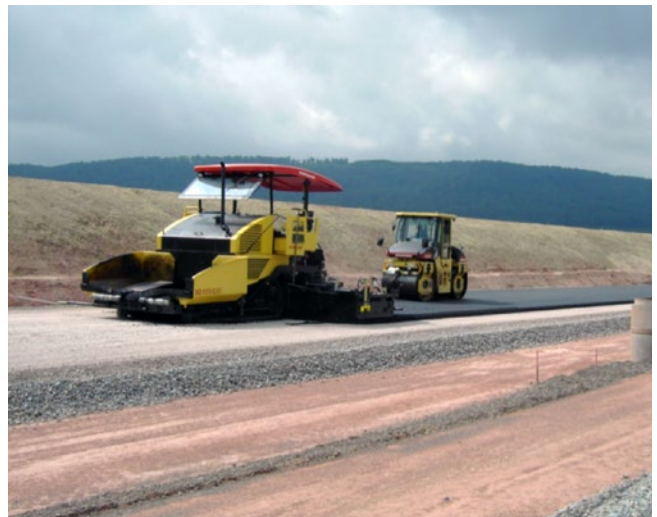
Figure 37: Prolonged interruption of paving due to inadequately planned asphalt mix logistics [11]
