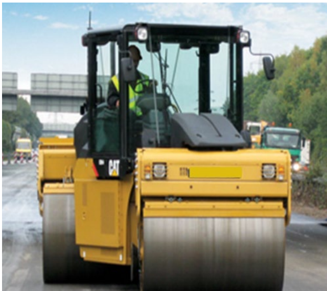
Figure 77: Final compaction with a tandem vibratory roller used for main compaction [7]
