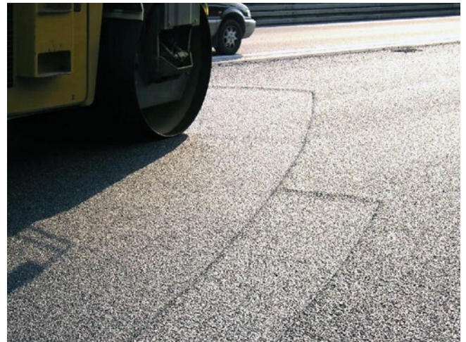
Figure 57: Elimination of the bow wave in front of the paving screed caused by the previous roller pass by means of a slight curve at the end of the following parallel strip [11]
