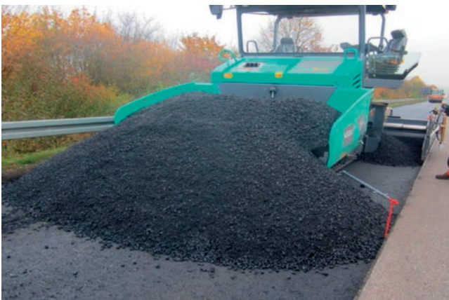
Figure 16: Paver stop due to improper material transfer to the paver [35]
