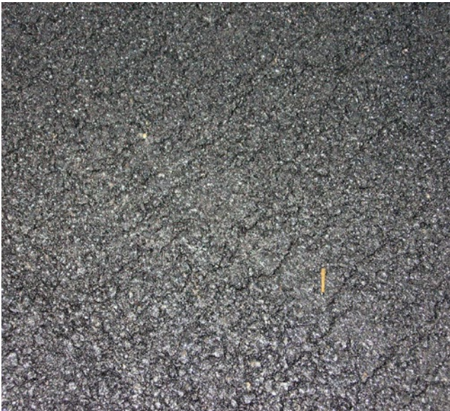
Figure 82: Transverse cracking directly behind the drum due to using a roller that is too heavy [11]
