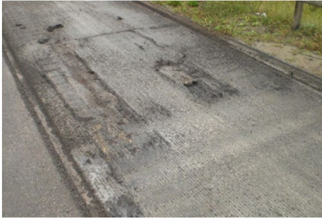
Figure 31: Imperfect surface and existing asphalt course after milling the asphalt surface course [7]
