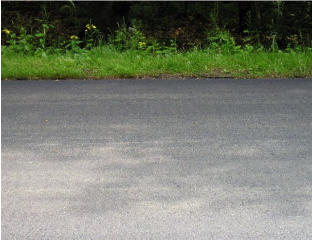
Figure 54: Formation of impact spacing marks due to excessive roller speed during vibration [11]
