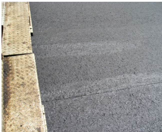
Figure 36: Condition of the SMA pavement as shown in Figure 35 after the incompletely cured bitumen emulsion has been paved over [11]
