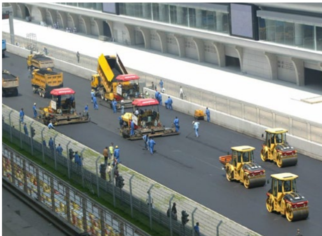
Figure 52: Variant of paving “hot to hot” with three pavers working in echelon [11]
