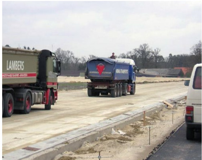
Figure 39: Identification of the vehicles delivering the asphalt mix for the surface course when laying a compact asphalt pavement [11]
