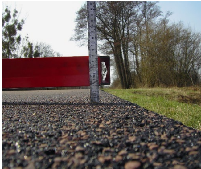
Figure 72: Formation of a shoulder due to incorrect rolling on the outside of an asphalt course that is unsupported [11]
