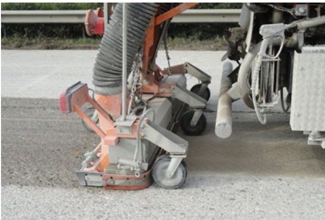
Figure 29: Cleaning a milled surface with a high-pressure rotary jet washer-suction unit [20]
