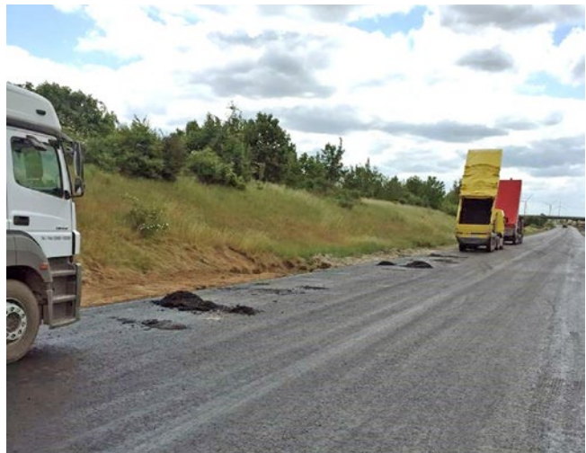
Figure 40: Negative example: Residual mix spread across the construction site after cleaning the truck loading rims [35]
