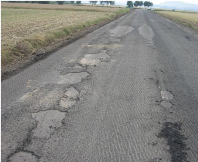
Figure 28: Scabbing and delamination on a milled base [11]
