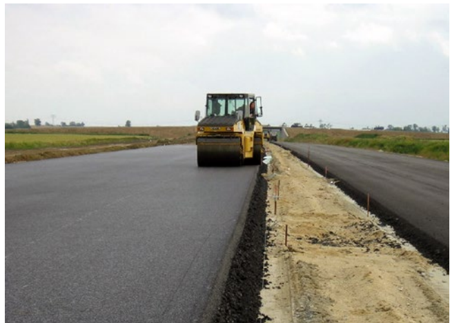
Figure 74: Gentle compaction of the unsupported edge of a paved asphalt course with the aid of crab steering [11]
